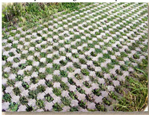
Fig.4 concrete grass pavers
