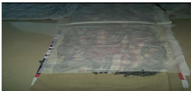
Fig 4. Efficient curing pad for curing to concrete
