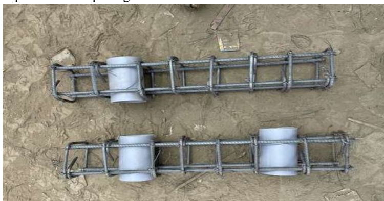
Fig 4.4.1 Reinforcement &amp; Openings
