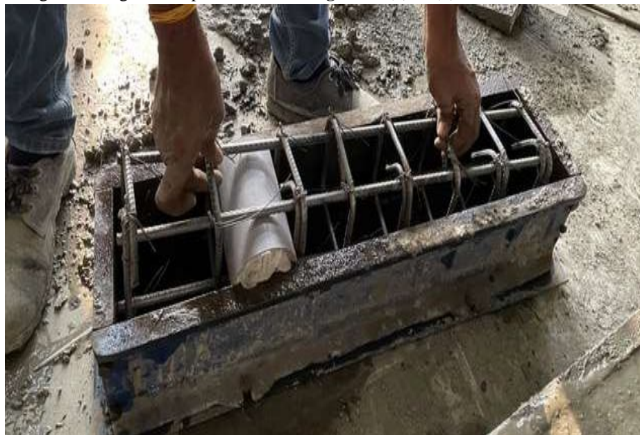
Fig 4.4.2 (a) Formwork
