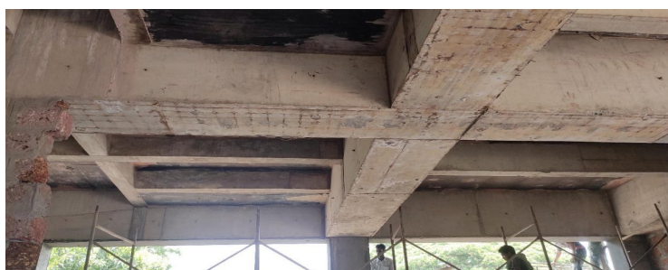
Fig. 3 Primary and Secondary beams in First Floor
