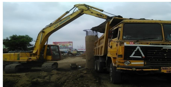
1.4 Loading in Tipper (Ashok Leyland)
