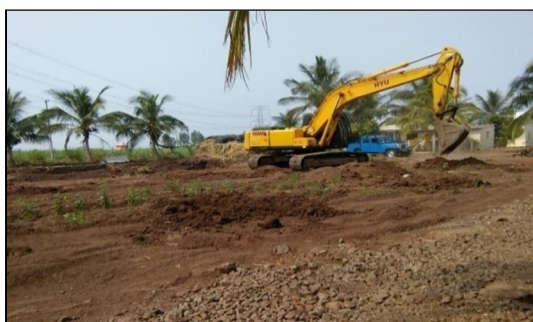
1.1 Excavation by Crawler type excavator-(HYU 220 LC-7)
