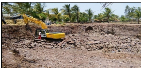
1.2 Excavation by Crawler type excavator-(HYU 220 LC-7)
