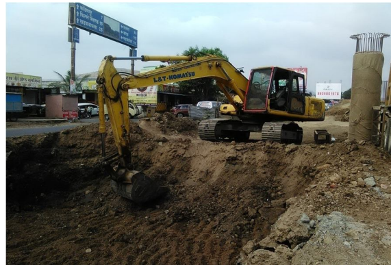
1.3 Excavator (L& T- Komatsu PC-200)
