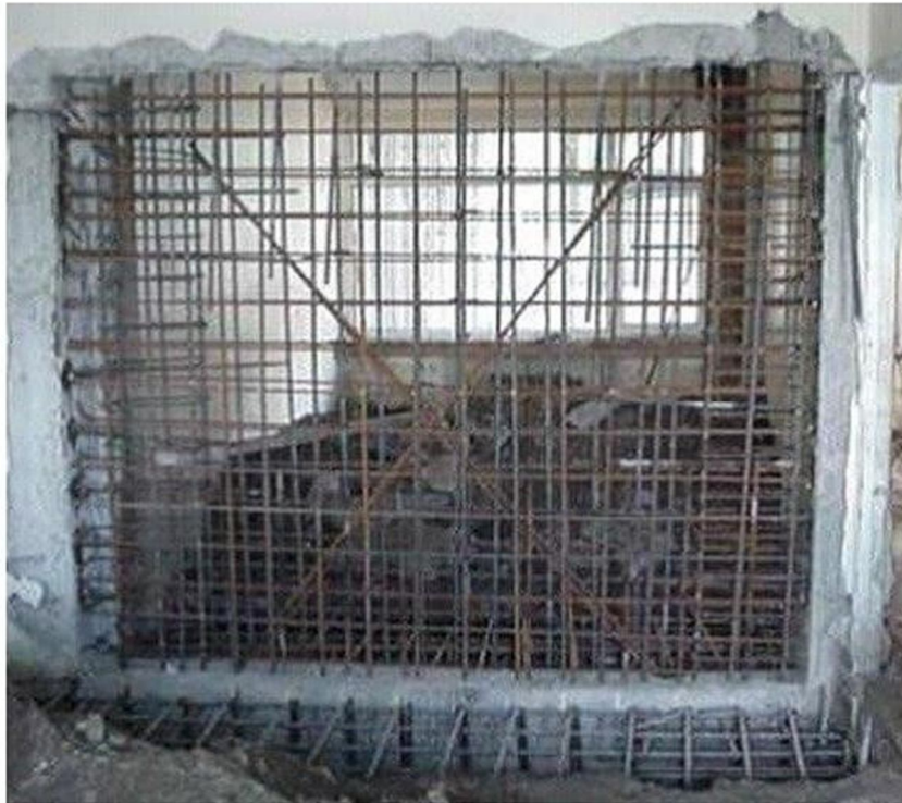
Fig 1.2. Additional Shear Wall
