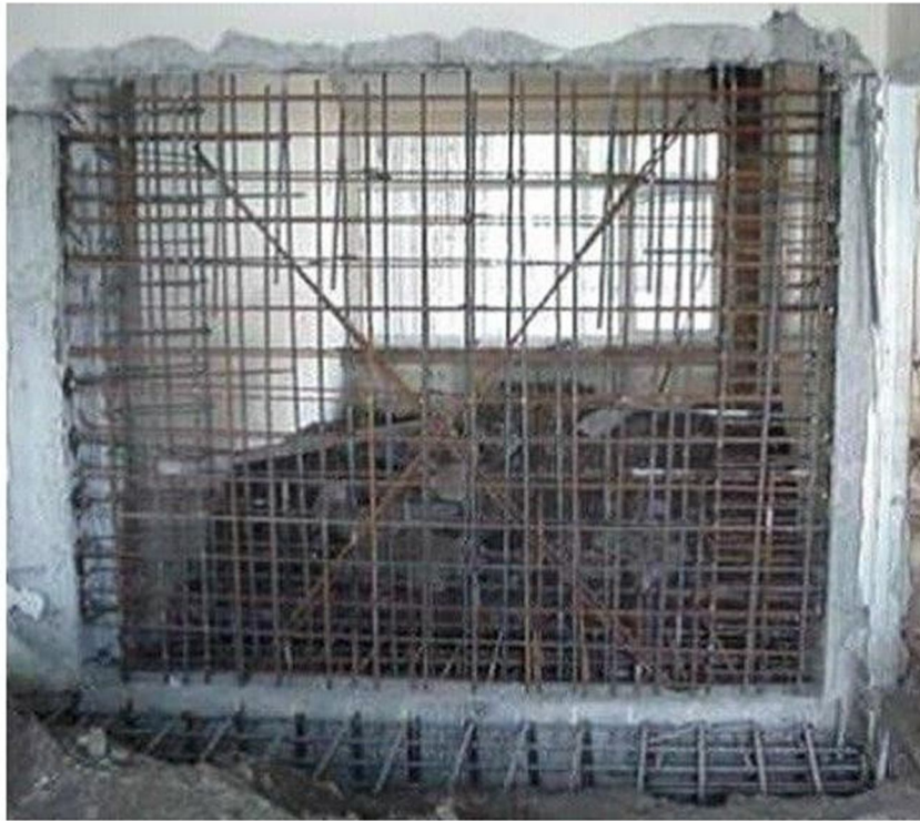
Fig 1.2. Additional Shear Wall
