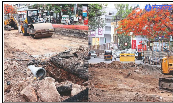
Fig. 2 Demolition of CBS to Canada Corner – Model Road
