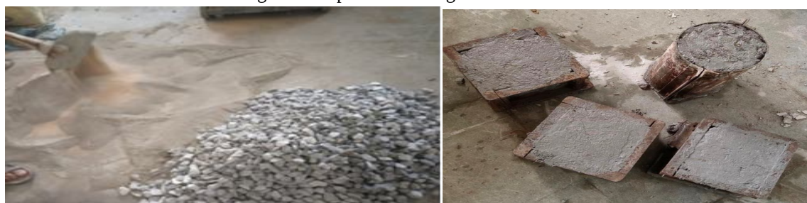
Figure: - Mixing of materials & Casting of specimen
