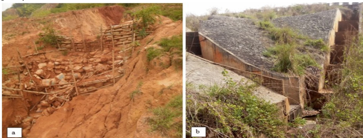
Fig.1.1: Different technical methods used mitigate soil erosion and slope failures in the biggest gully site in South eastern (Nigeria): (a) sand bags (b) runoff breakers (Igwe and Una 2019).
