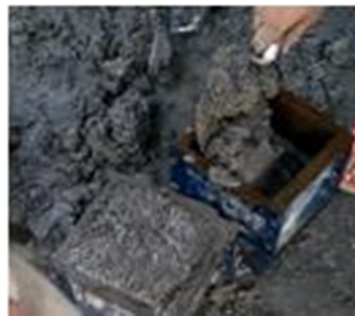
Figure 3: Filling mortar in moulds
