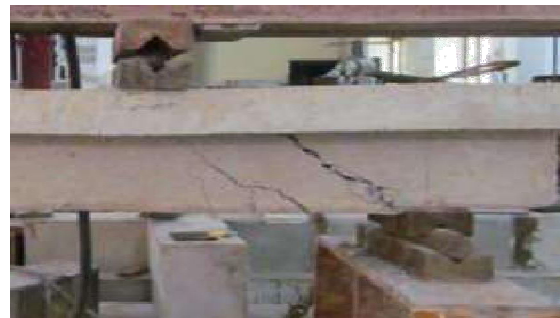
Fig 4 Widened crack at ultimate load
