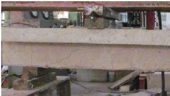
Fig 3 Hair line crack started at 110kN
