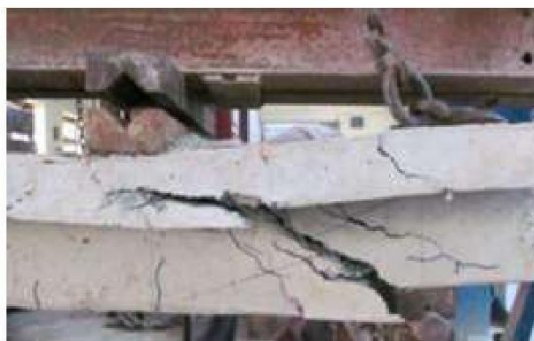
Fig 7 Widened crack at ultimate load
