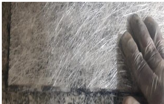
Fig 3 : Layer-02- Chopped Stranded Mat layed over layer-01
