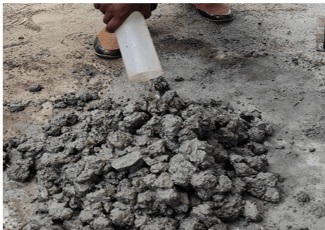
Fig 4 Mixing with Admixture
