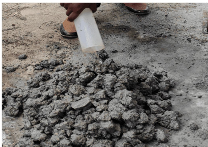
Fig 4 Mixing with Admixture
