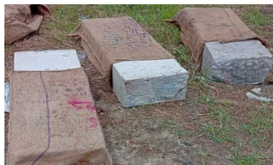
Fig 15 Curing of Beam
