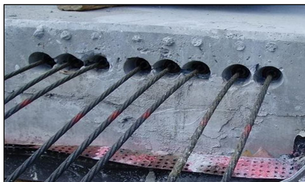
Fig.2 Tendon (cable) tails after tensioning
