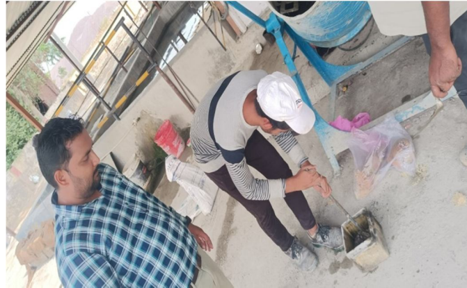
Fig.4.4: Compaction with Tamping bar
