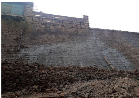
(c) Horizontal grouting from dam d/s 2c
