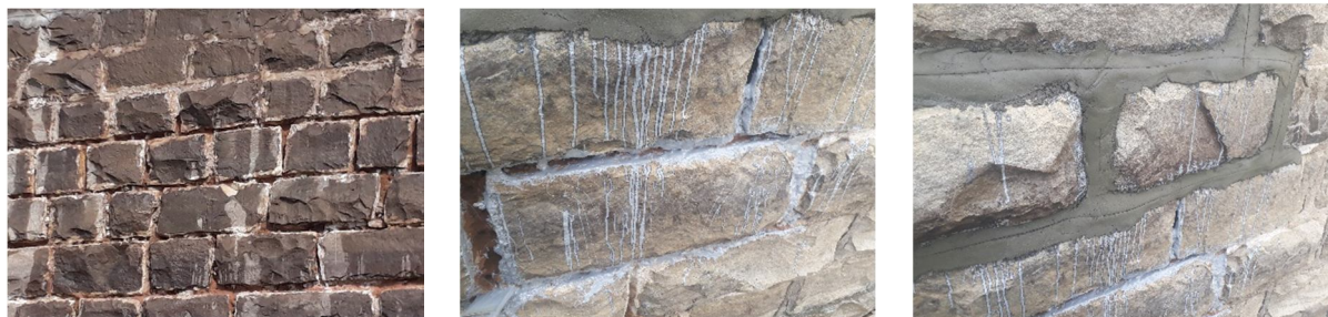
Fig.3 Different stages of surface preparation
