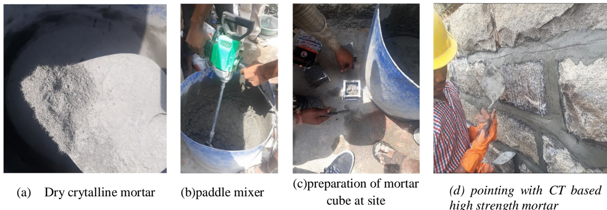
Fig.3 Application process of high strength mortar)
