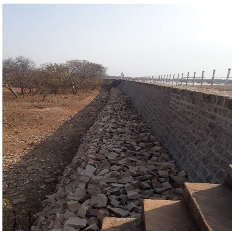
(a) Construction of Gabion wall 2a
