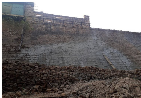
(c) Horizontal grouting from dam d/s 2c
