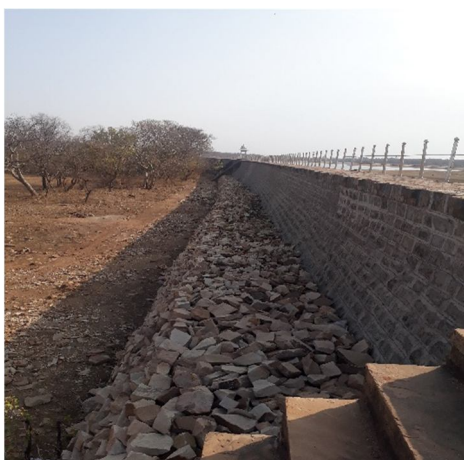
(a) Construction of Gabion wall 2a
