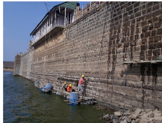
(b) Surface preparation at dam u/s 2b
