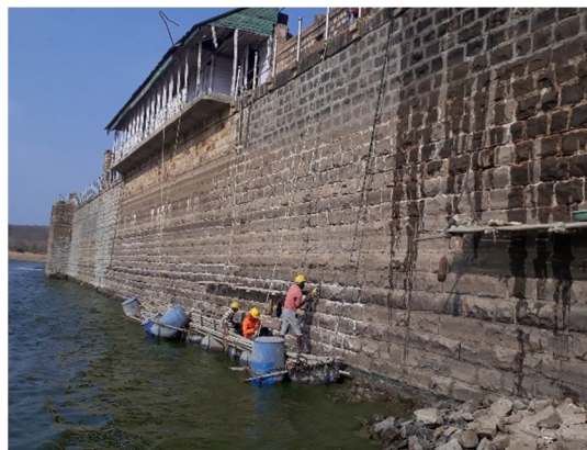
(b) Surface preparation at dam u/s 2b
