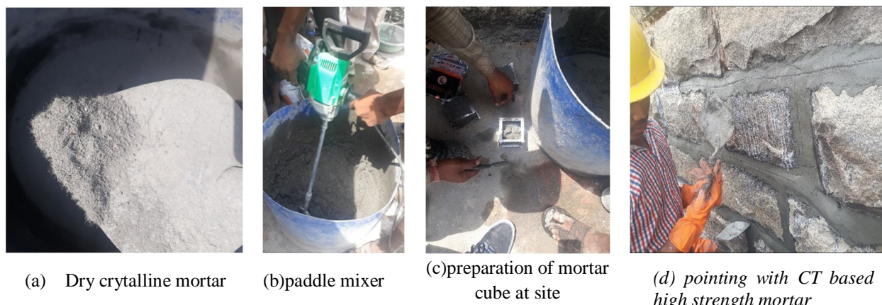
Fig.3 Application process of high strength mortar)
