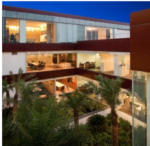
Fig.2: India Glycol Campus (source: archdaily.com)
