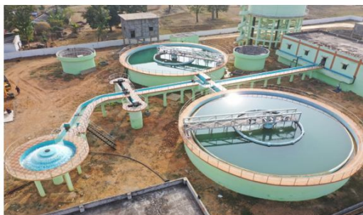
Figure-5-Clariflocculators
