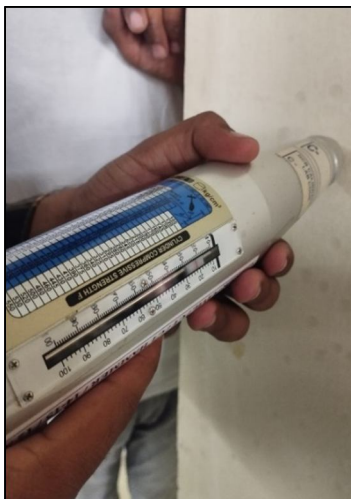
Fig. 4. Rebound Hammer Test
