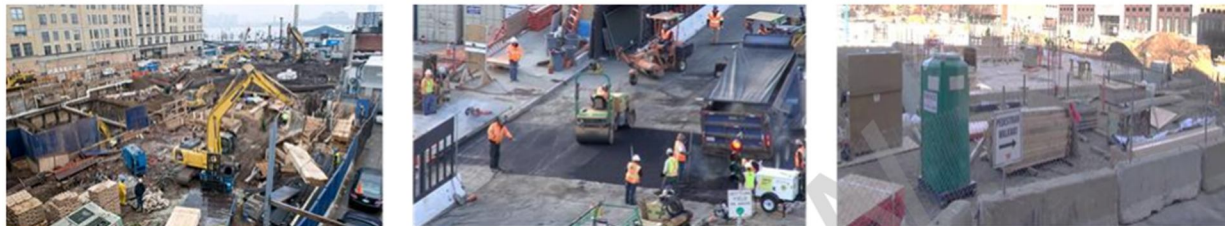
Figure 1: Examples of complex and unstructured construction sites
