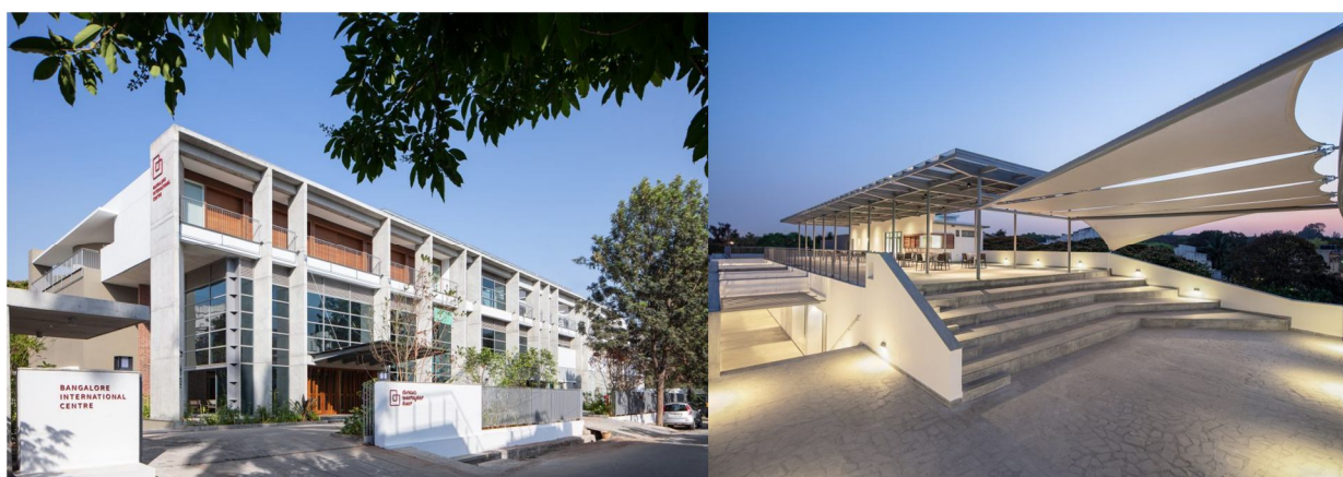
Figure 12 Bangalore International Convention Centre (Source: Photo Gallery - Bangalore International Centre )
