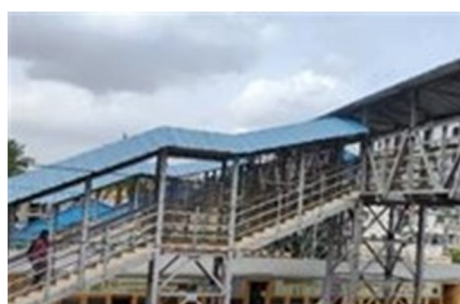
Figure 22: Foot over bridge in railway junction
