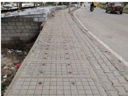
Figure 13: Good & Useable footpath Condition Source: Author
