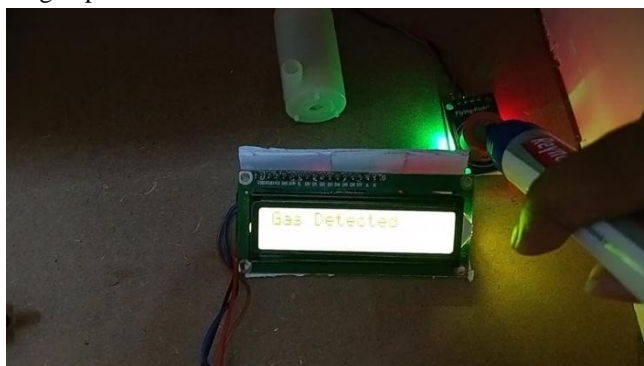
Fig. 12. Gas leakage detection and warning system
