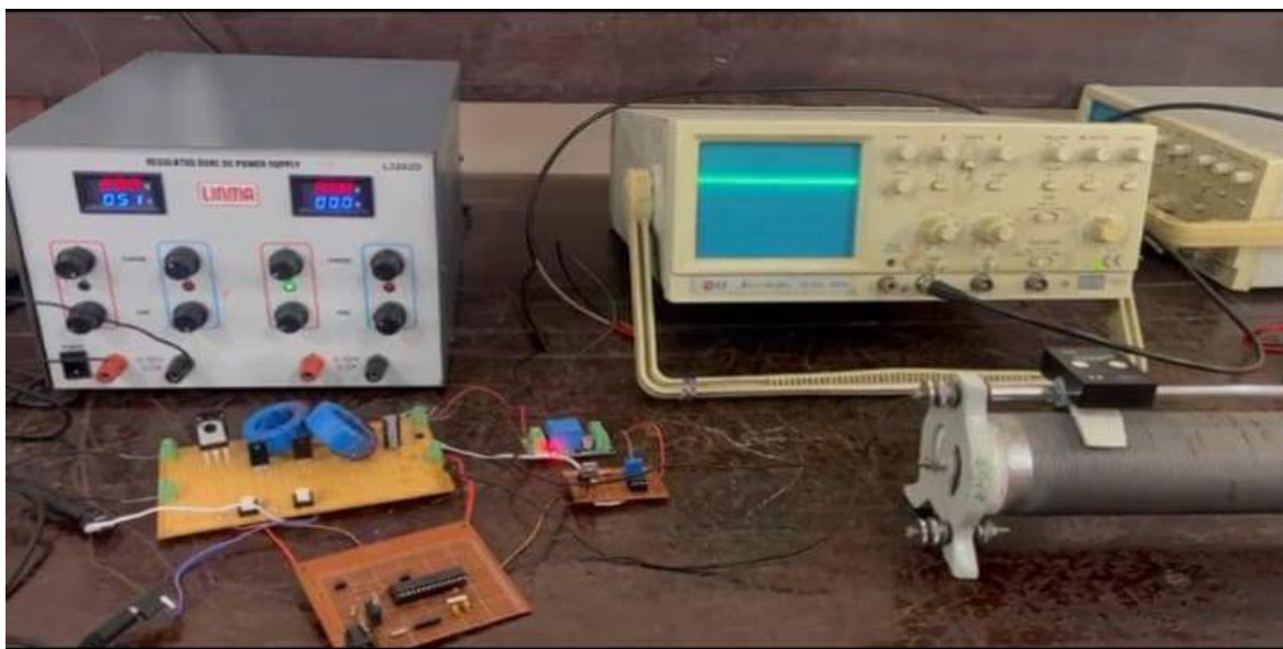
Figure 6 Hardware setup of IBC with overvoltage protection
