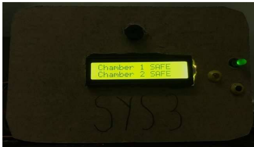
Figure 11.1 Sprinkler system during clean air scenario
