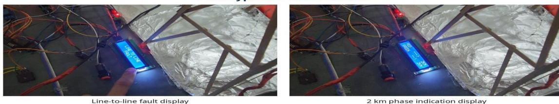
Figure 2. Prototype LCD and phase indicator observations during fault simulation Table 3 showing cloud-recorded current values, fault tag, distance and GPS coordinates.
