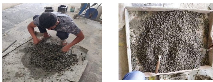
Figure 3.1 : Mixing of Pervious Concrete
