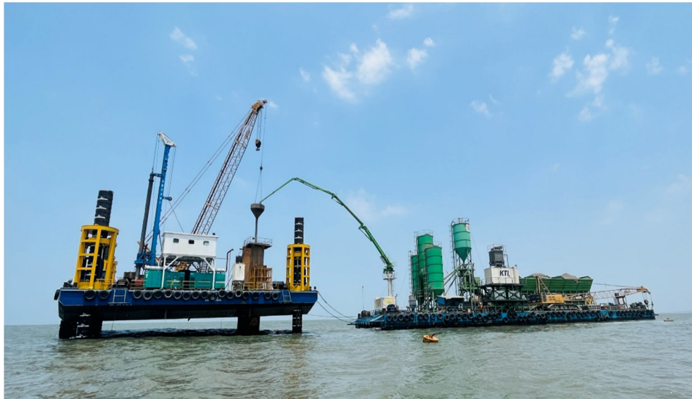
Fig-8: Pile Concrete pour with Floating batching plant
