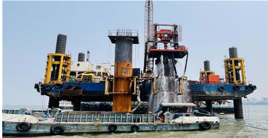
Fig-6: Jack up barge Drilling by RCD
