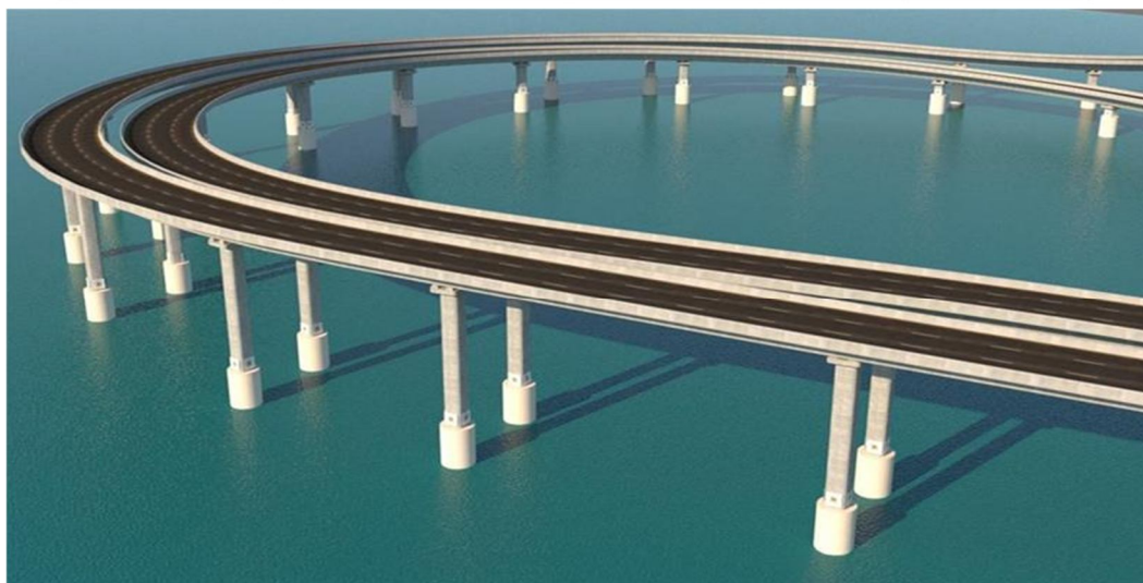
Fig (3): Aesthetic view with Monopile Foundation.
