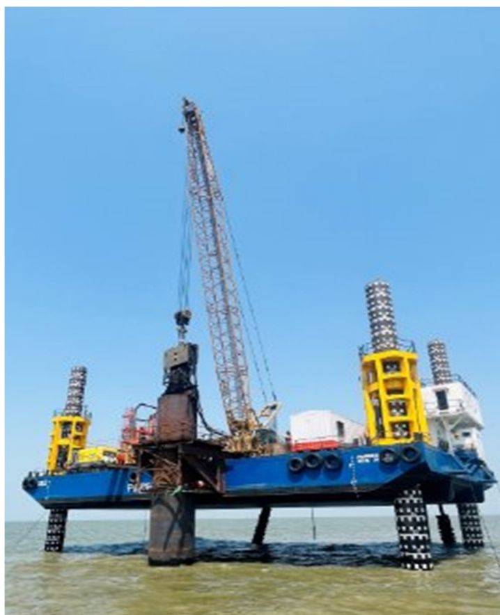
Fig-5: Liner driving with Vibro-hammer
