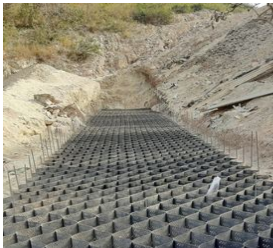
Figure1: High density polyethylene geocell laid for construction.
