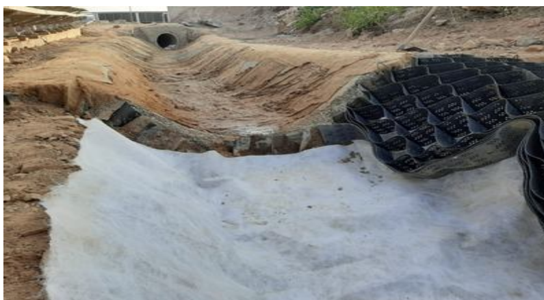
Figure 2: HDPE Geocell along with non-woven geotextile membrane
