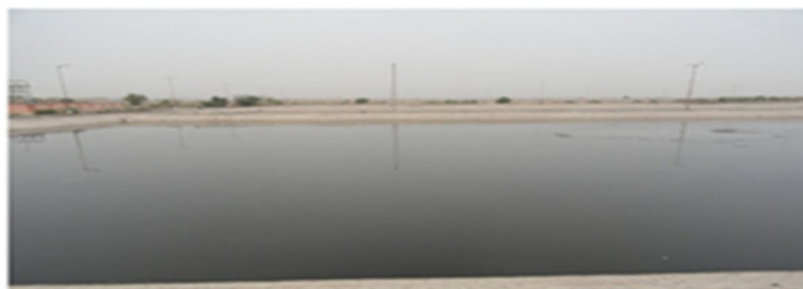
FIRST ANAEROBIC STABILIZATION POND, BIKANER
