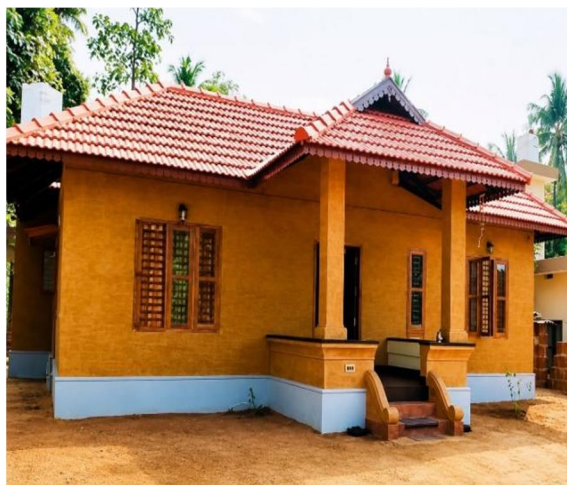
Figure 1: Mud-plastered house. (Chiluka, S.) 2023
