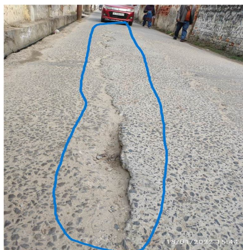
Figure 14 Pot holes at tuns
