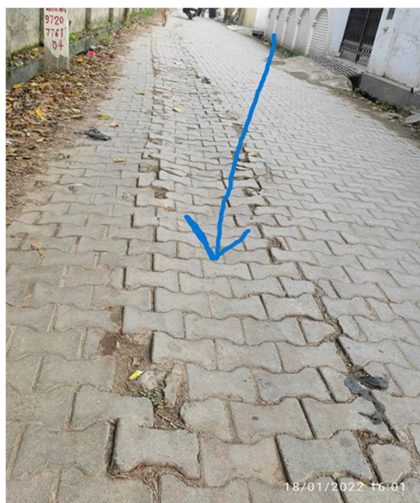
Figure 7 Interlocking Bricks Roads Settlement
