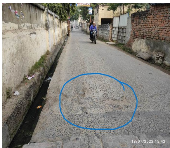
Figure 13 Eroded encasement surfaces
