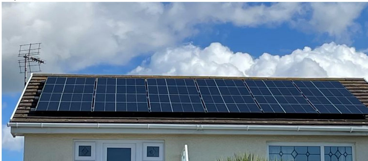
Figure 1: Optimal condition for installation of solar panel
