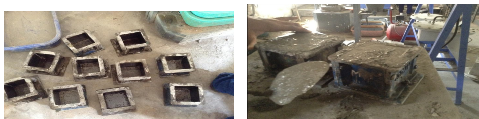
Fig –3.3 casting of cubes.
