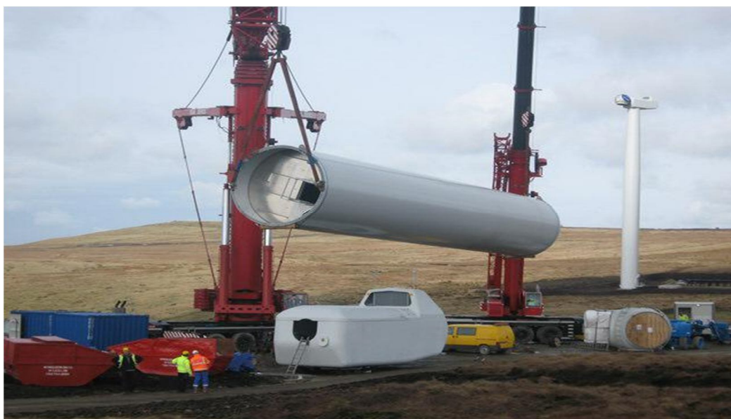
Figure.1. OSH risks associated with the construction of wind turbines (Unloading of Tower cells)
