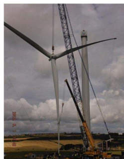
Figure.2.Erection of Tower cells & Blades
