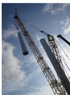
Figure.2.Erection of Tower cells & Blades
