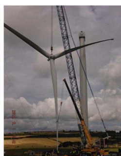
Figure.2.Erection of Tower cells & Blades
