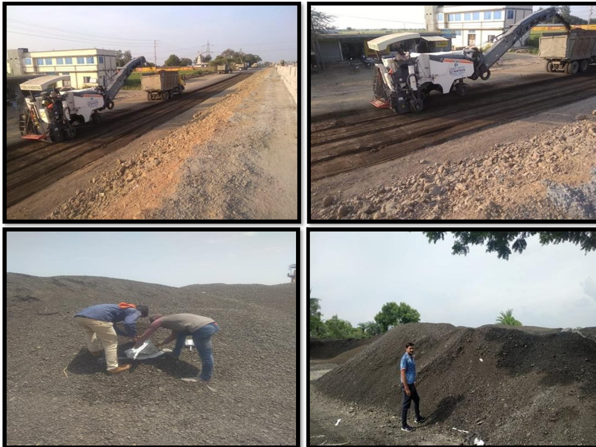
Figure-: Milling of existing bituminous layer at site & Sampling of material from stockpile
