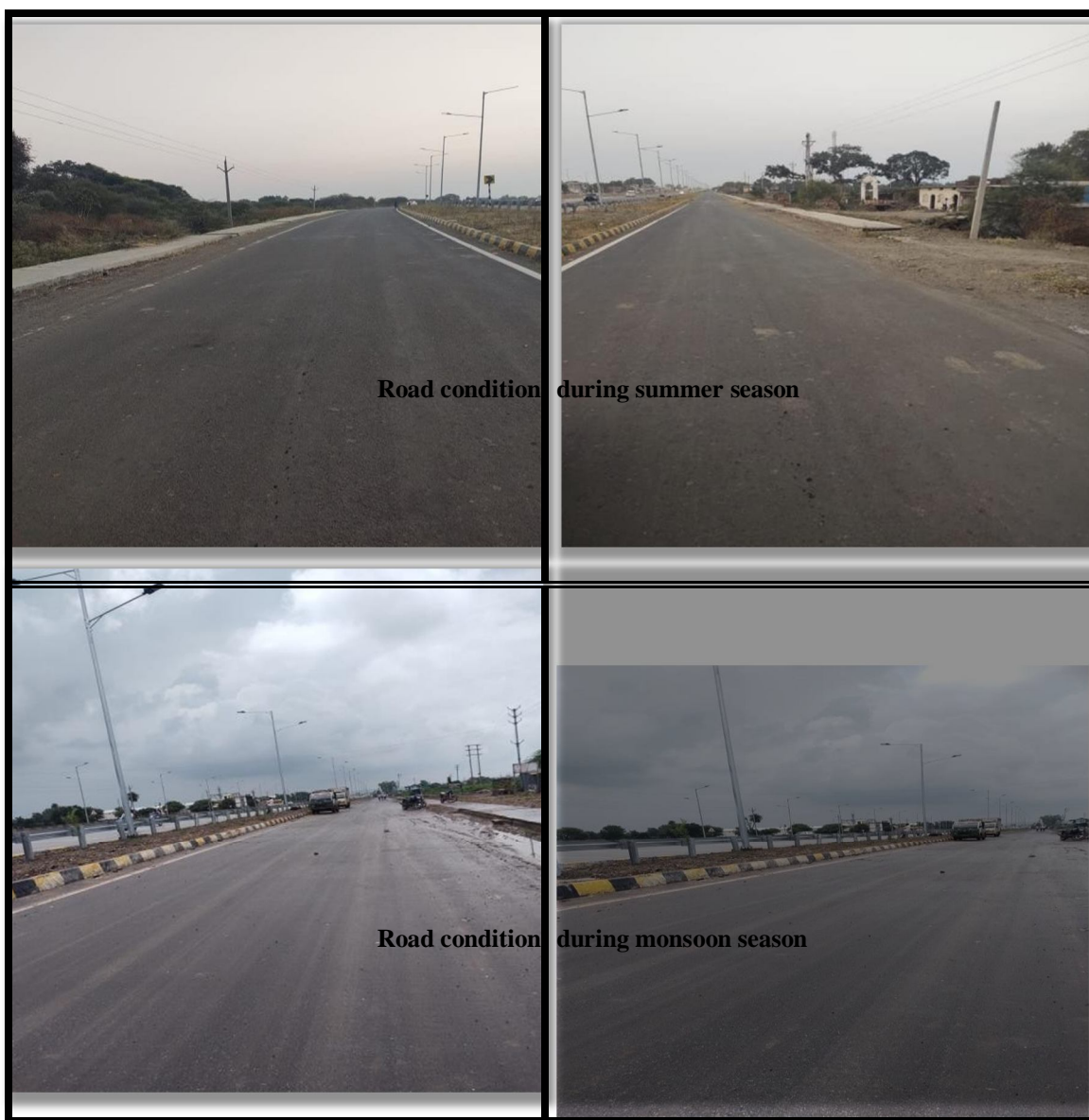
Figure:- Serviceability of various weather condition
