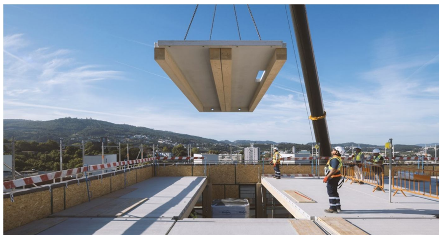
Figure 1 – Assembly of the B&B Hotel Guimarães modules.
