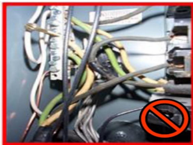
Fig no: 4.1 Exposed Electrical Parts
