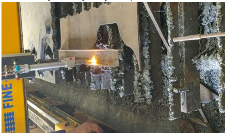
Fig. 6 Castellation Process (Cutting of I-beam using CNC machine)
