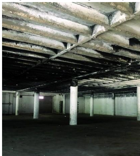
Figno.1FireDamageBeam
