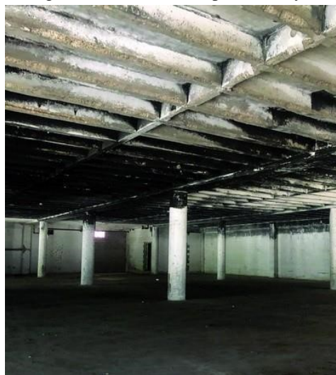
Figno.1FireDamageBeam
