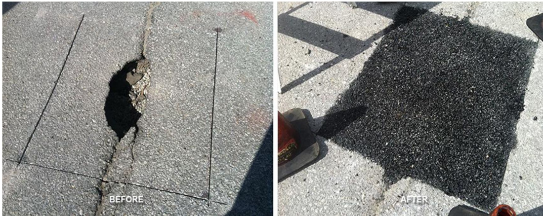
Figure 3.4: Before-and-After Photographs of Repaired Sections in Pratapgarh and Chilbila.
