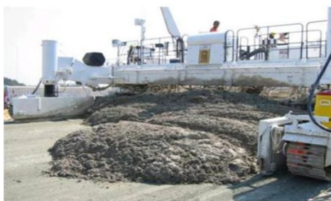
Fig. 1. Concrete mixing plant
