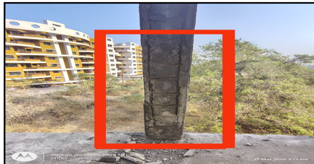
Photo 2) Spalling of concrete from Column
