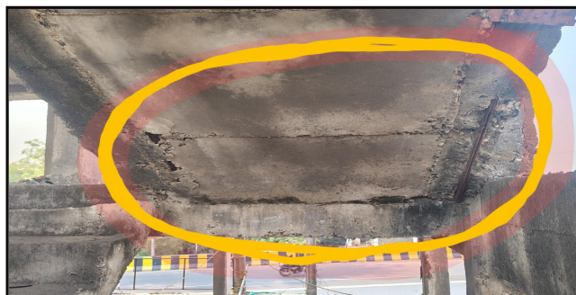
Photo 1) Reinforcement came out of concrete
