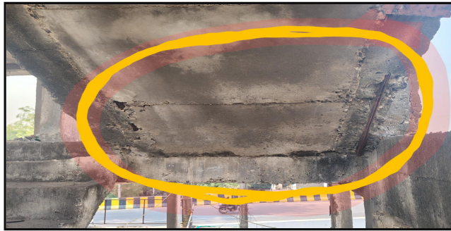
Photo 1) Reinforcement came out of concrete
