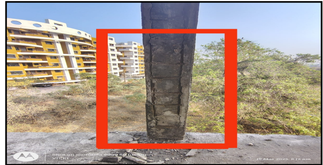
Photo 2) Spalling of concrete from Column
