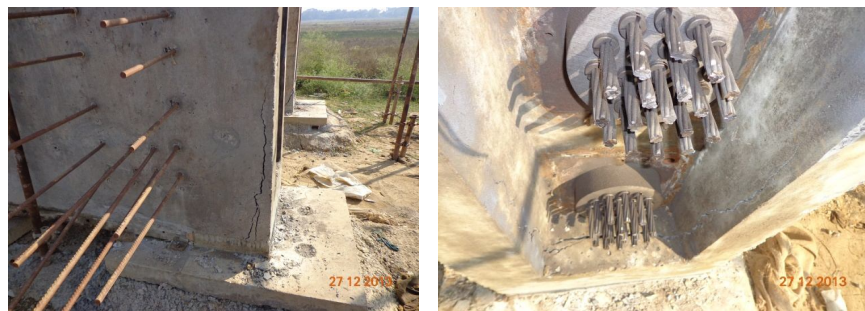
Fig 4.1:- Removal of Girder Concrete skin due to Rigid casting bed at End Block portion.
