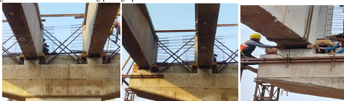
Fig 1.3:- Supporting arrangement of PSC Girdes (3 Photos)
