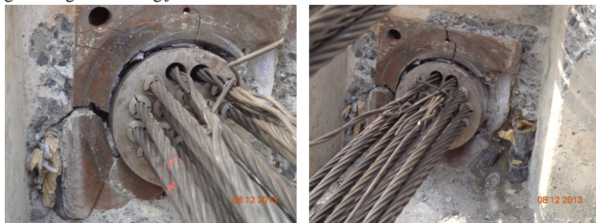
Fig 2.1:- Failure due to cavitation & grouting ducts (Anchor Cone Puncture)
