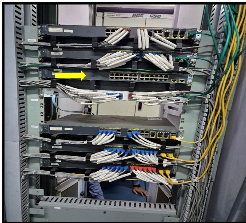
Above is New Network Switch installed (CISCO Catalyst 9200 ) for Status Monitoring of NET-A and B for DCS
