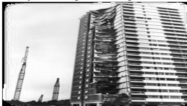
Fig. 1.1: Ronan point building after 1968
