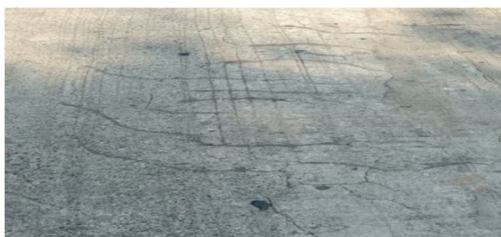
Plastic Shrinkage Cracks
