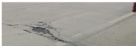
Spalling at cracks
