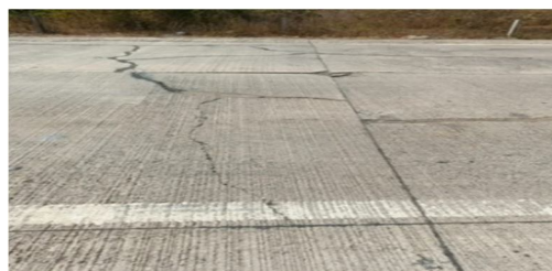
Transverse Cracks
