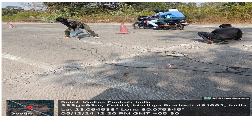
Fig.4 Filling of joints using bitumen sealant
