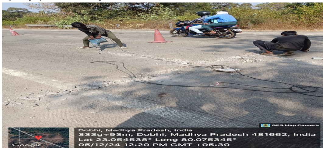
Fig.4 Filling of joints using bitumen sealant
