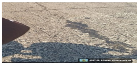
Loss of surface Texture, polished surface
