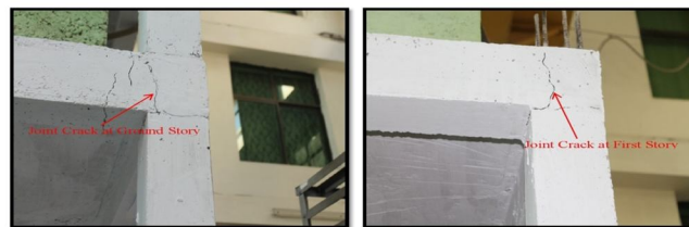
Beam-Column Joint Crack at Ground Story
