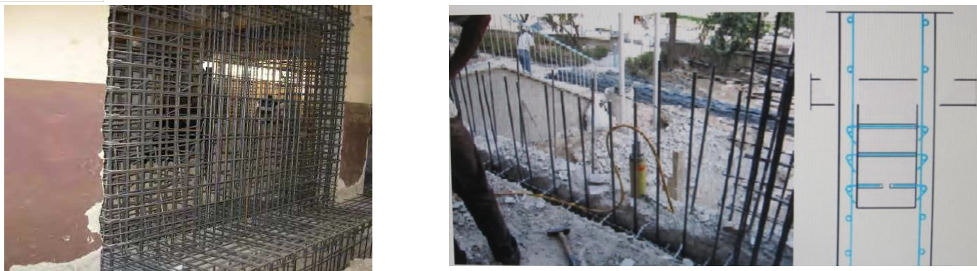
Fig. 2 System based strengthening of RC members
