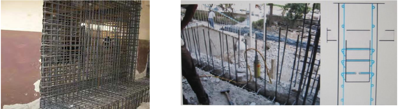
Fig. 2 System based strengthening of RC members
