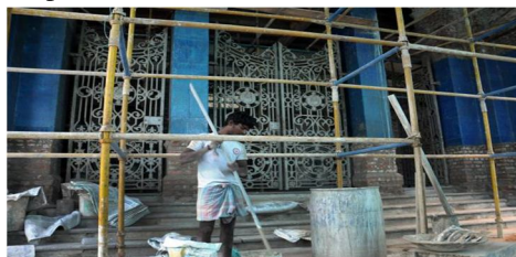
Fig4. Wrapping the Chennai Corporation Building with Fibre
