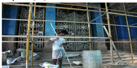
Fig4. Wrapping the Chennai Corporation Building with Fibre
