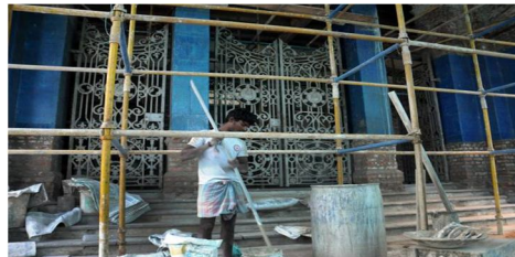
Fig4. Wrapping the Chennai Corporation Building with Fibre
